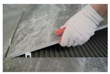
These flexible joints are inserted along all areas where the tiles meet the building and across the floor at intermediate spacings. Your tiler must also use an adhesive suitable for the type and size of tile and the expected temperature fluctuations to prevent tenting.
